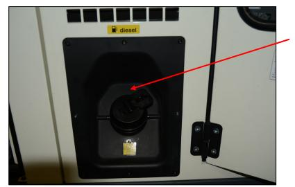
To begin installing the wiring harnesses, remove the diesel fuel inlet assembly shown here by removing all the screws around the perimeter and loosening the hose clamp on the back side.
