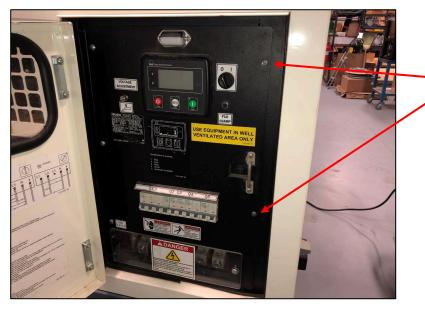
Remove two (2) electrical panel bolts (the electrical panel can now be swung open).
