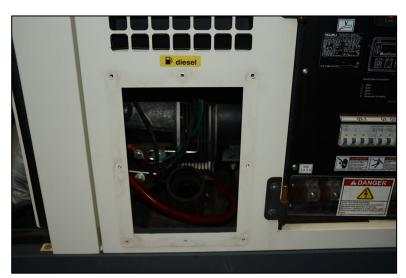
Here, the diesel fuel inlet assembly is shown removed. There is a neck down into the fuel tank that will need to be covered using either a plastic bag or plug to keep debris from contaminating the fuel.
