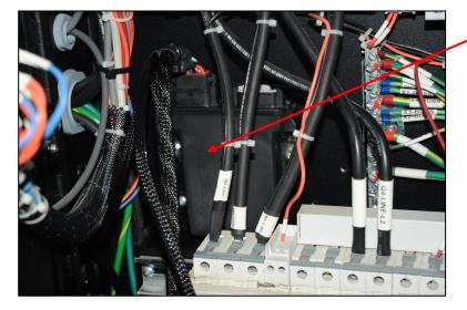
Verify there is nothing on the rear side of the control box that will be damaged, and then using the two selfdrilling screws included, mount the controller in the location shown here.
