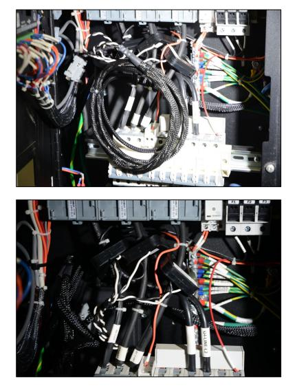
Back inside the electrical enclosure, attach the 3 current transformers to the cables passing through the existing current transformers (grey objects at top of photo) making sure to encapsulate <u>ALL</u> wires passing through the existing wires. Make sure to match labels on the Ventech supplied current transformers with the current transformers already in the enclosure. From left to right, these should be "U", "V", and "W".
