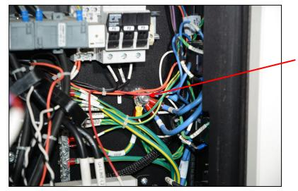
Locate the breakers labeled "F1", "F2", and "F3" in the upper right corner of the electrical cabinet. Loosen the top 3 screw terminals and terminate the 3 stripped voltage sensing wires as shown. From left to right, this should be brown (U), black (V), and purple (W). Retighten screws and verify both the sensing wires and the existing wires are both held securely in the terminals.
